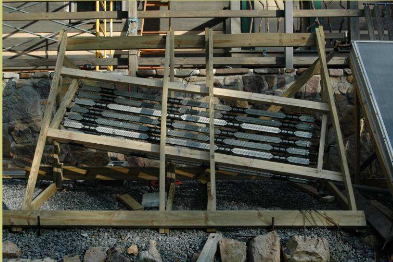
Figures 1, 2. Heat Dump (baseboard radiant tubing).
